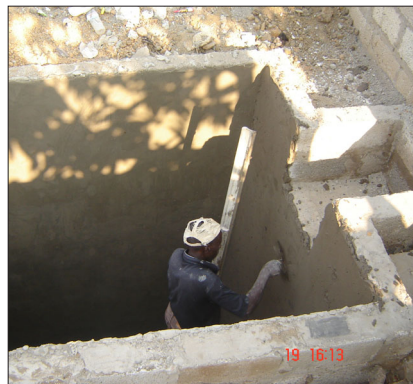
Building the Septic Tank
